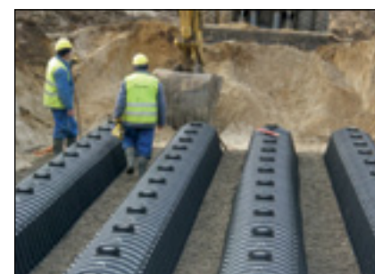
Zona industrial, Raben (PL)
